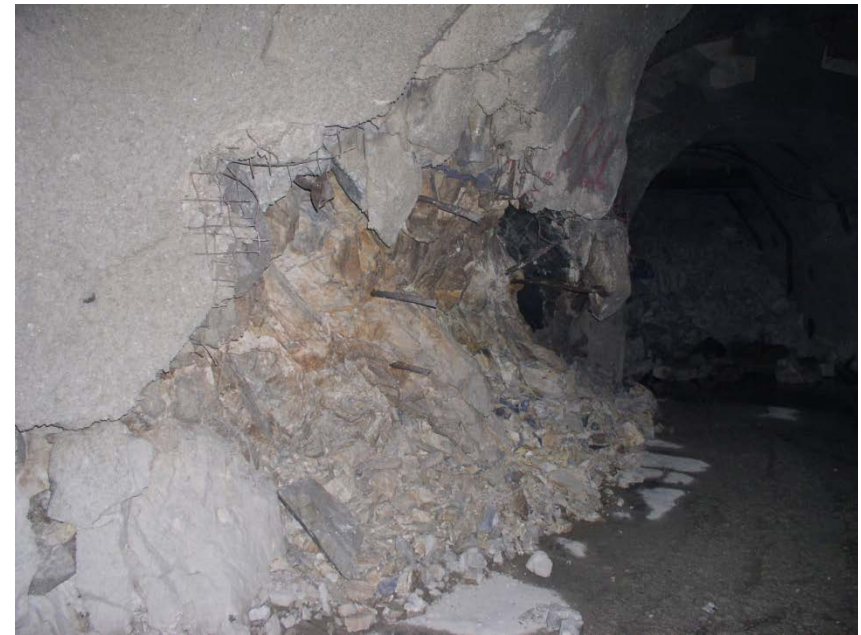
Slabbing at the side of opening (production level)
