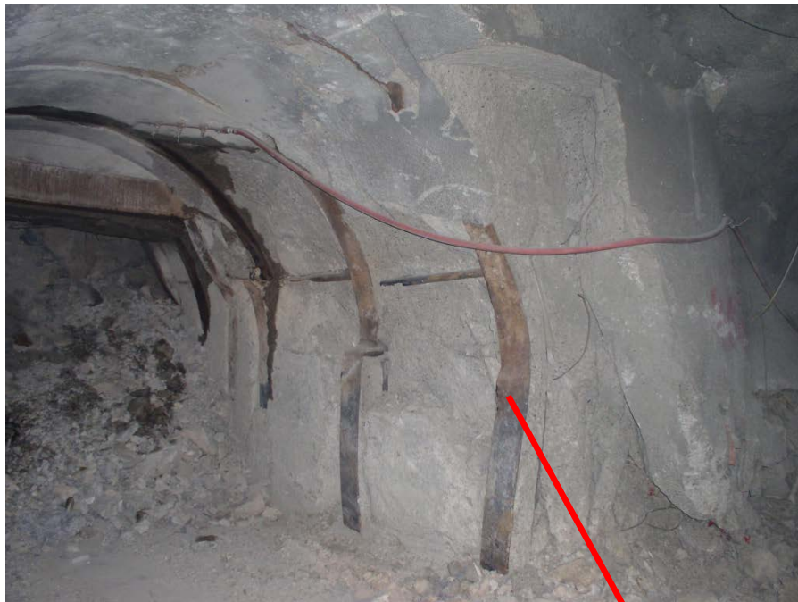
Defected steel rib 휘어진 강지보
