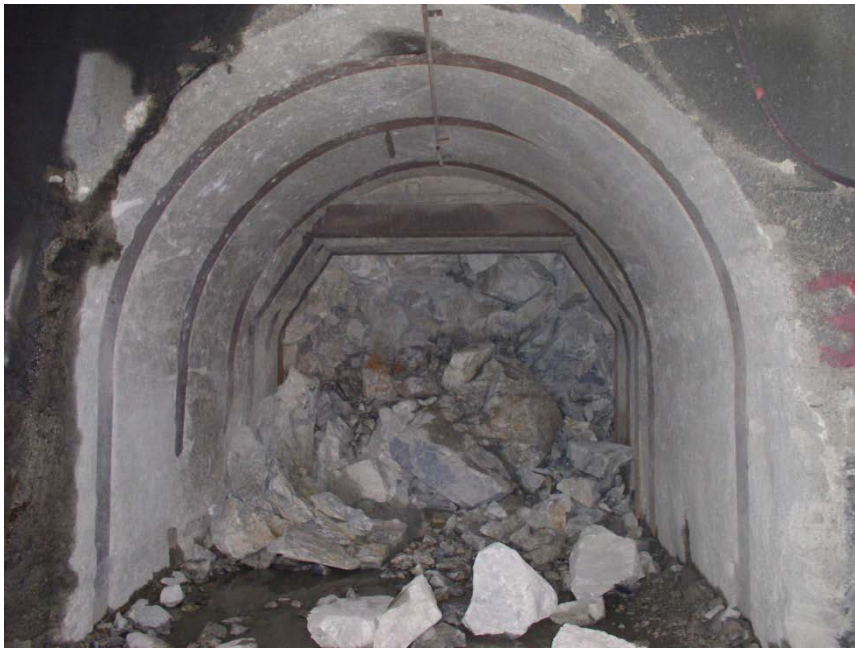
Relatively large ore size and intact concrete lining
