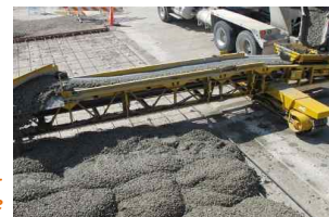
A belt conveyor to place roller-compacted concrete
