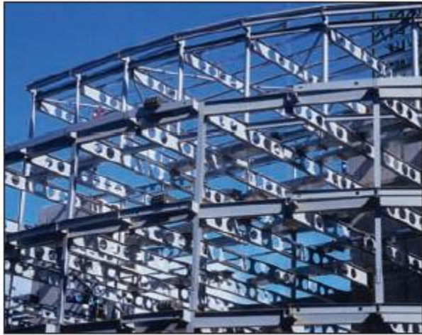
Nonprismatic beams with cutouts in their webs
