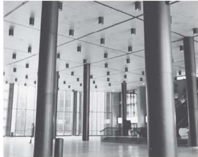
Fig. 16.34 The array of large, cylindrical, surface-mounted downlights dominates the area's appearance despite the high ceiling.
