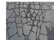
Map Cracking
