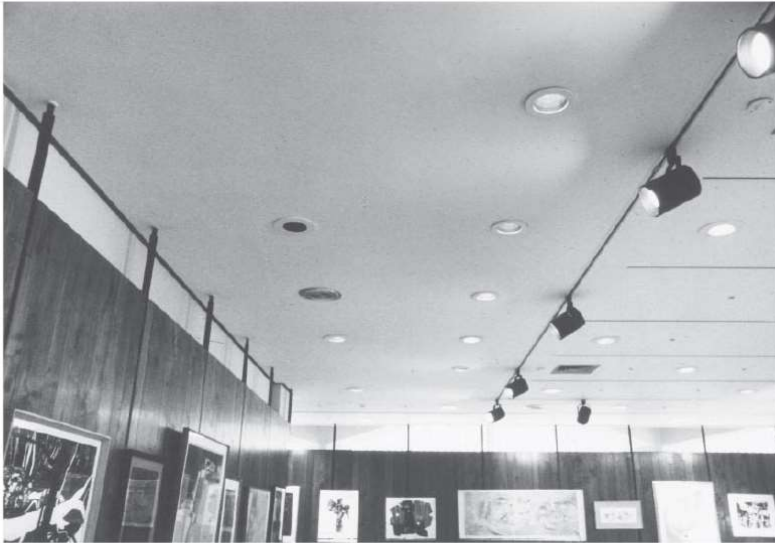
Fig. 17.9 Art exhibition room illustrating good and bad lighting techniques. The upper wall fenestration is excellent for deep daylight penetration. Track lighting is ideal for display of art. The use of incandescent downlighting for general lighting is excessive and an eyesore. Also, the positioning of the track fixtures can create both direct and reflected glare problems and annoying shadows unless the sources are selected properly and ceiling height is at least 10 ft (3.1 m).
