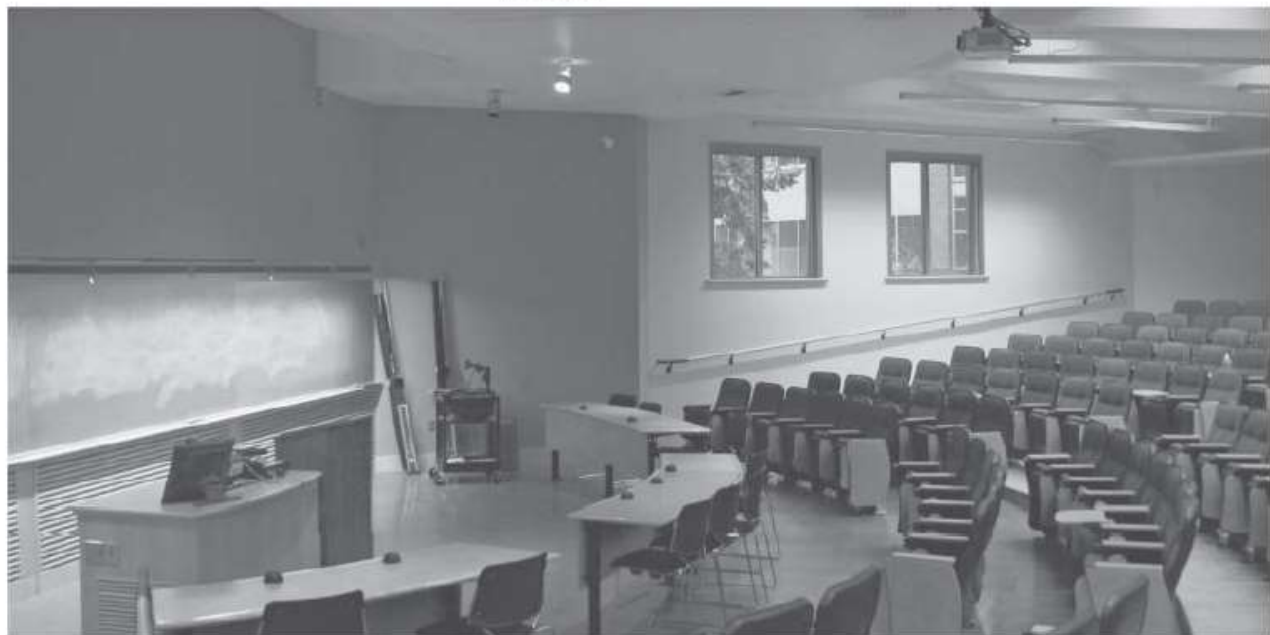
Fig. 17.12 Typical lecture room lighting utilizes 45° cutoff baffled parabolic reflector troffers for minimum direct and reflected glare, adjustable track lighting for demonstration table illumination, and an asymmetric reflector for chalkboard lighting. The large display area on the front wall of the room will not experience veiling reflections with the illustrated lighting arrangement.
