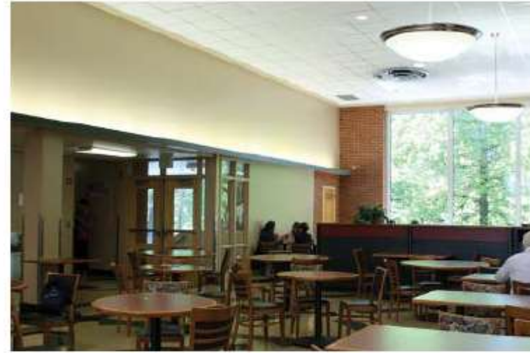
Fig. 17.11 Institutional cafeteria illuminated by cove lighting and daylight, accented with downlights and suspended pendants in a double-height space. Lighting is even, glare-free, soft in quality, and pleasant, yet of sufficient intensity to permit using the cafeteria as a working-meeting space. (© Karen Tse; used with permission.)
