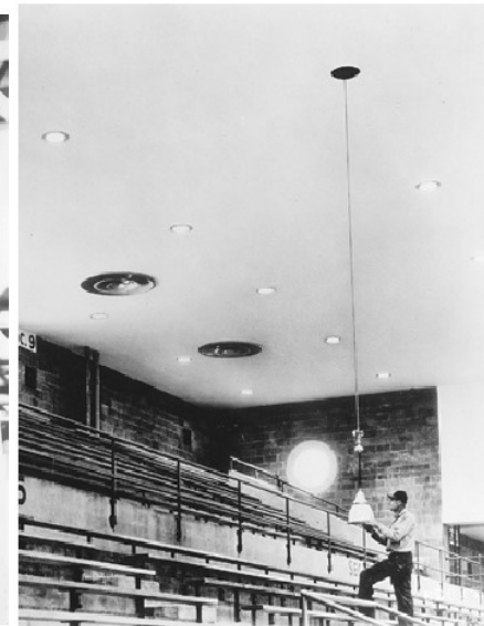
relamping from the floor
