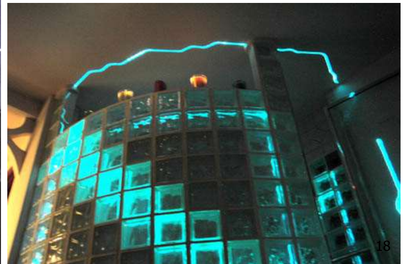
Fig. 17.33 Side-light-emitting FO cables are ideal for linear lighting tasks such as stair-edge illumination, under-shelf lighting, and outline lighting of all sorts. The illustrated 3-tail arrangement is representative of this type of FO lighting.
