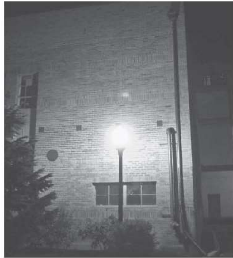
Fig. 17.29 A "lollipop" fixture, even if aesthetically pleasing to some, gives poor illumination downward (note the large collar). This type of luminaire causes light pollution. (Photo by Nathan Majeski.)
