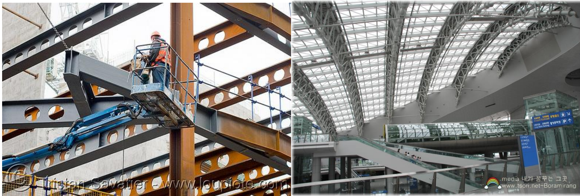
Steel frame of building
