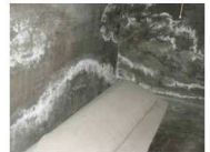
Efflorescence
