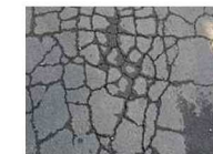
Map Cracking
