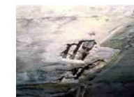
Corrosion of exposed rebar
