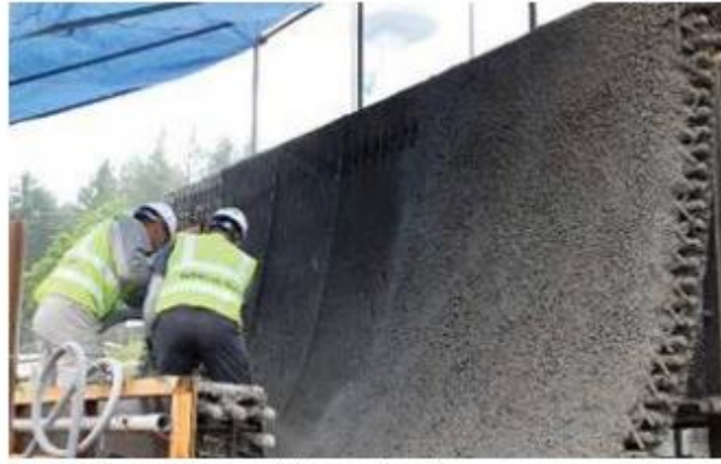
Fig. 5: Shotcreting the sliding track wall
