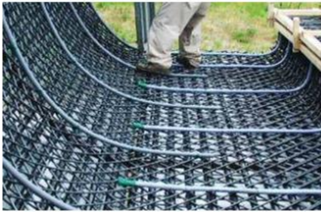
Fig. 4: Track section ready for shotcreting
