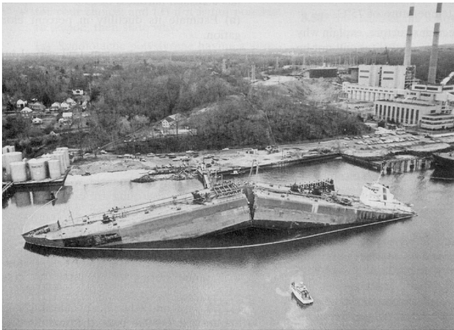
Oil tanker fractured in a brittle manner
