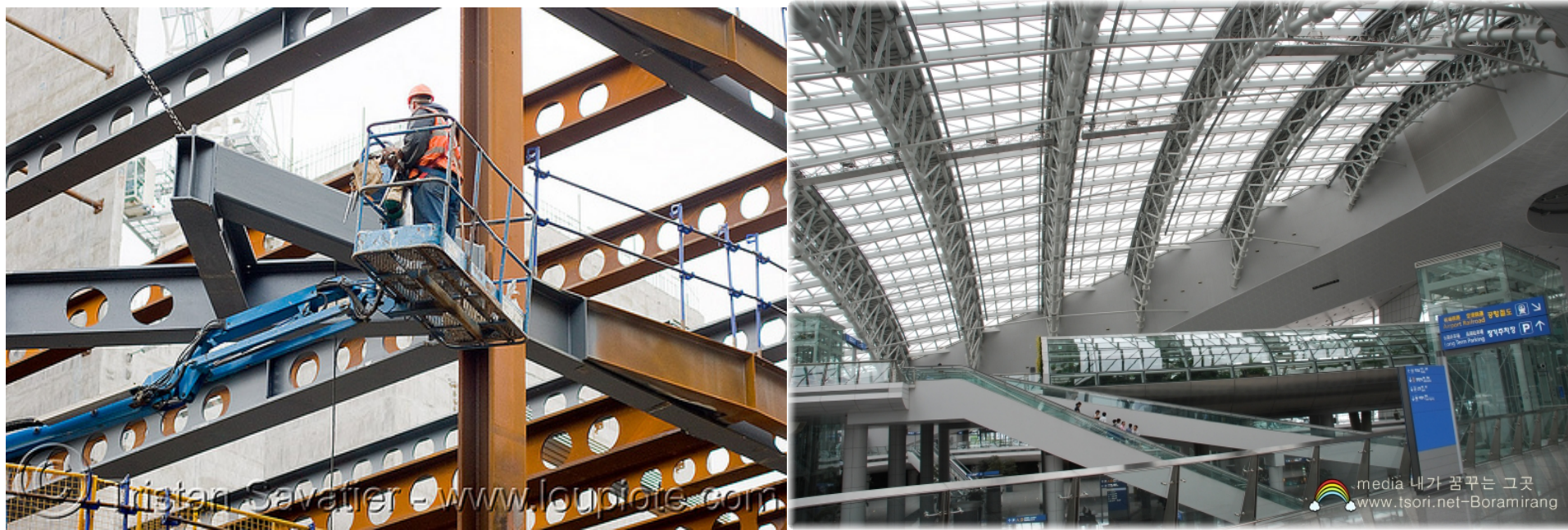
Steel frame of building
