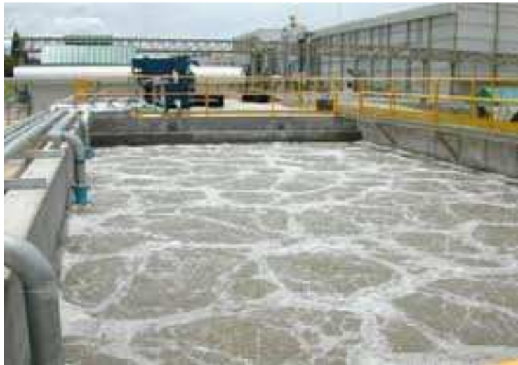
Biological wastewater treatment
