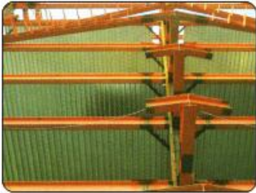
Steel frame of building
